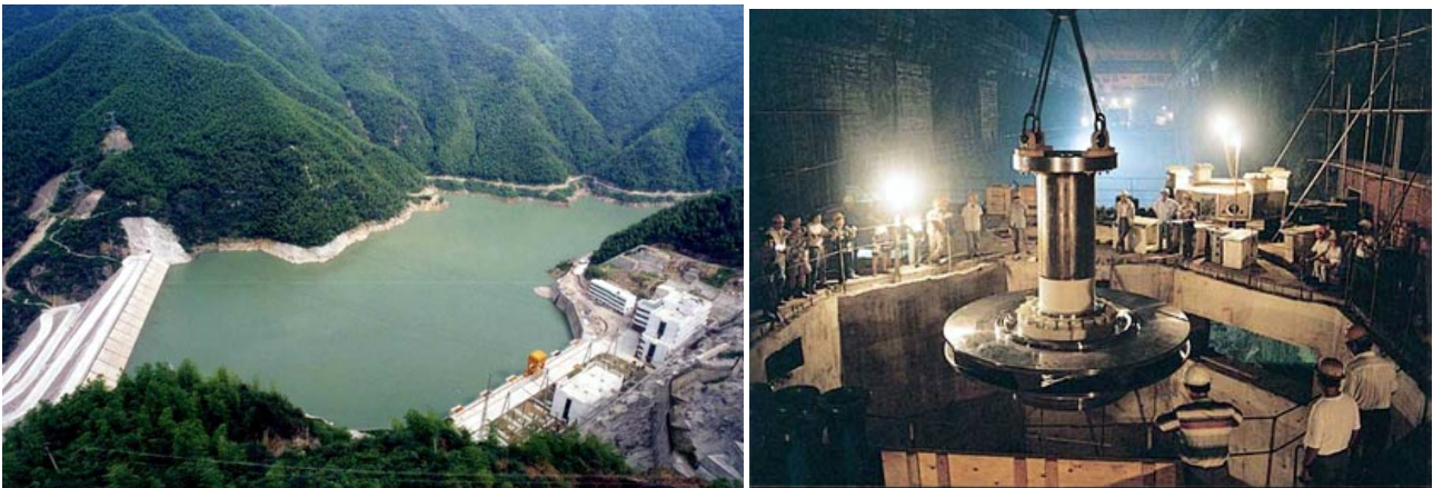
Figure 8. Tian Huang Ping Lower reservoir (left picture) and installation works (right hand side) (Ref. Wikipedia)
